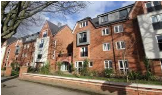
Oakfield Court, Urmston
